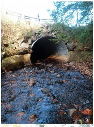
1. The culvert is getting crushing from the pressure of route above.
