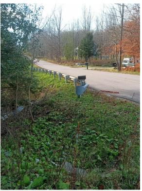
3. The digital level shows how French Hill Road is settling over the culvert.
